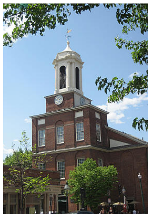
Canback Dangel's office at the Charles Street Meeting House 121 Mount Vernon Street, Boston
